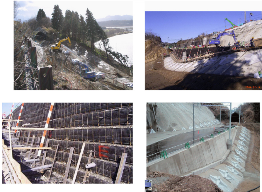
Fig. 22. Reconstruction to a GRS-RW with a full-height rigid facing, site 1 (cf. Fig. 20b).
