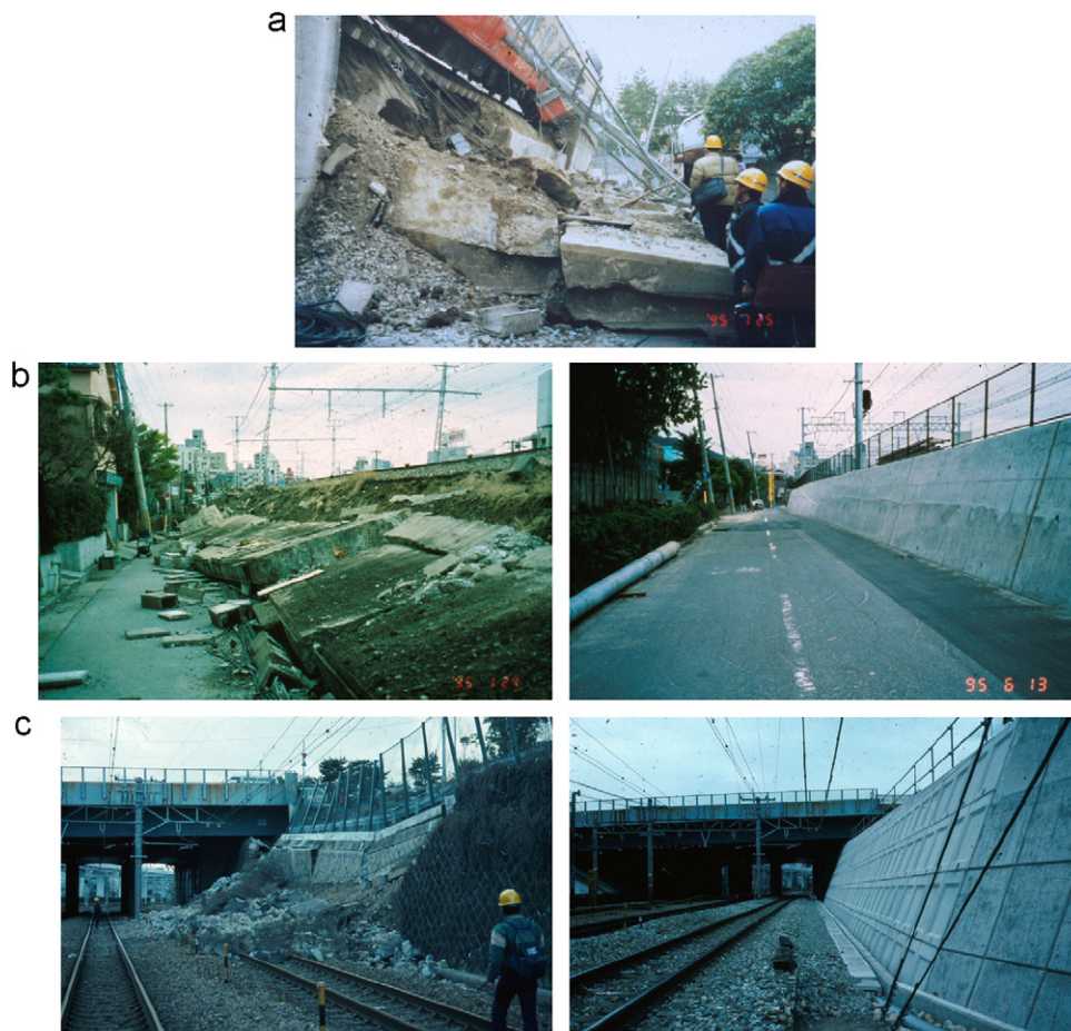
Fig. 14. Typical damage to conventional type RWs; (a) gravity-type wall at Ishiyagawa Station, Hanshin Line (site G1 in Fig. 13); and (b) and (c) gravity (leaning type) and masonry walls (sites L1 and MS1 in Fig. 13) and reconstruction to GRS-RWs with a full-height rigid facing at Sumiyoshi, JR Kobe Line.
