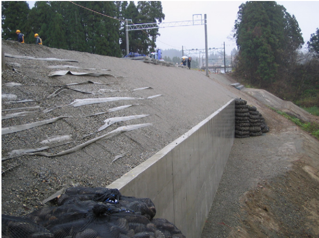
Fig. 24. Reconstruction to a GRS-RW with a full-height rigid facing, site 3 (cf. Fig. 21b).
