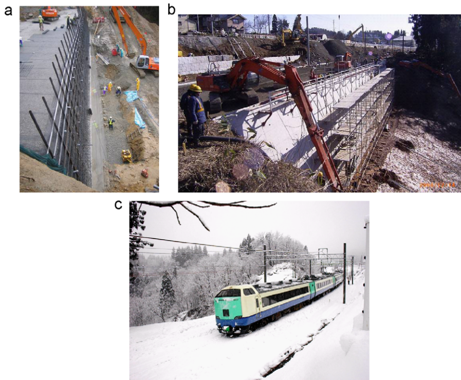
Fig. 23. Reconstruction to a GRS-RW with a full-height rigid facing, site 2 (cf. Fig. 19b).
